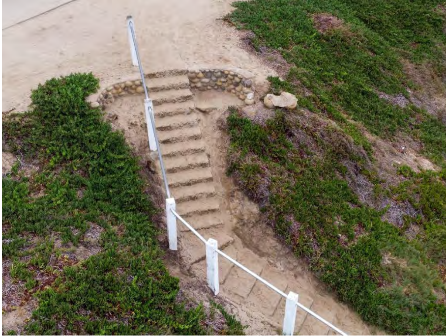
Photo 33 Whale View Point Stairs, camera facing south
